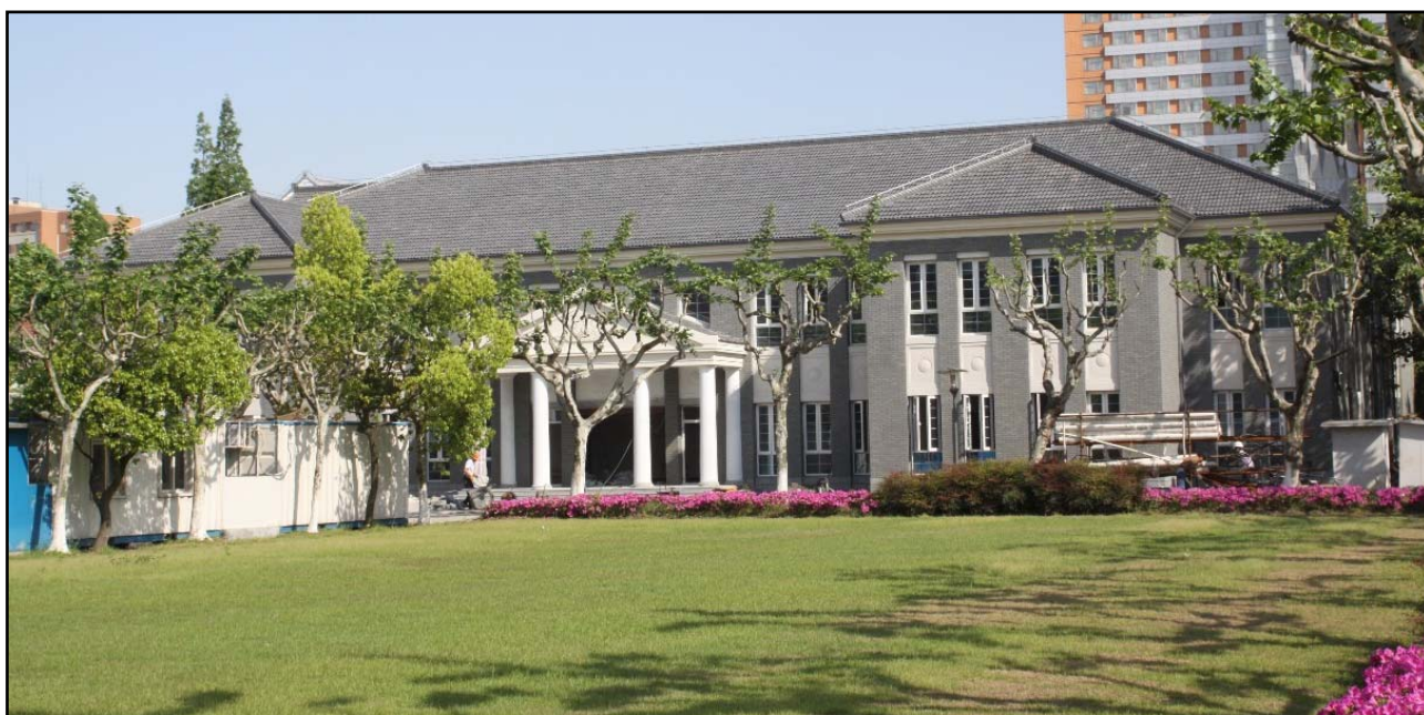
The New Nordic Centre building at Fudan Campus, picture from May 2010 when the building was in the final construction phase.
